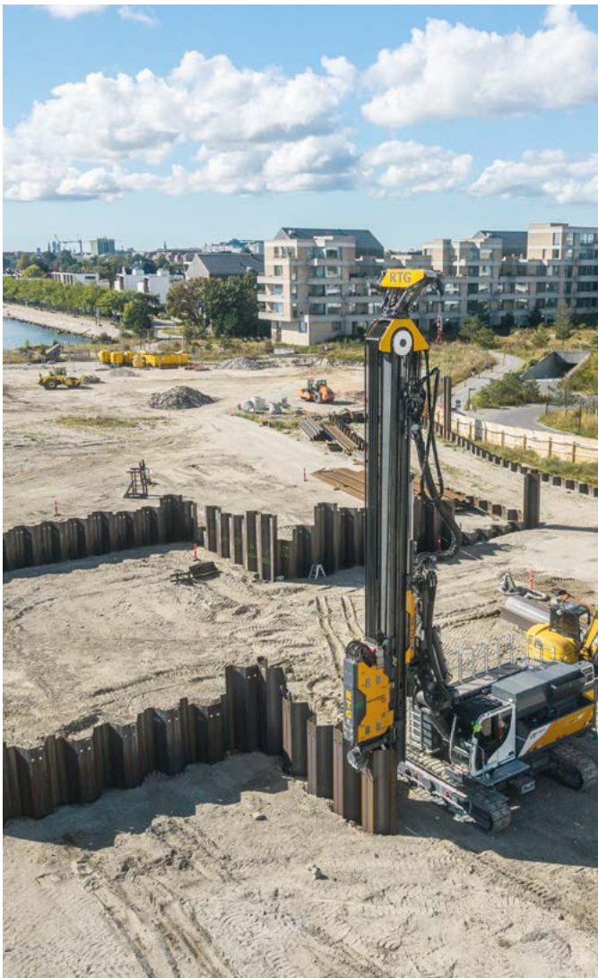
Spundwand-Rütteln Sheet Pile Vibratory Driving
