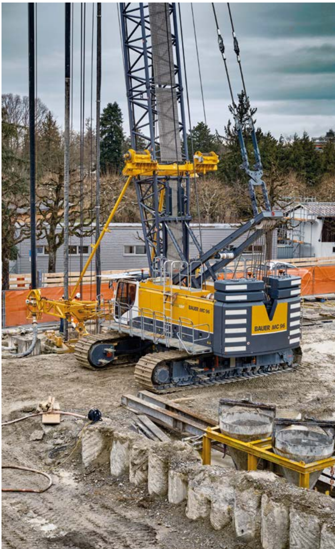
Gefräste Schlitzwand Diaphragm Wall with Cutter
