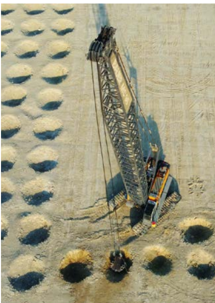
MC 96, Baugrundverbesserung, Abu Dhabi MC 96, Soil Improvement, Abu Dhabi
