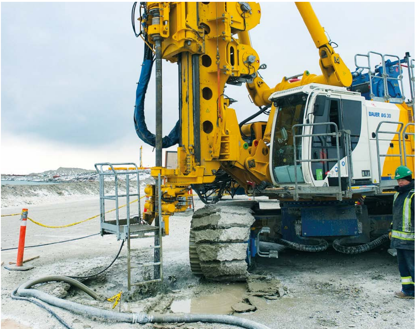
BG 30, Dichtwand, Kanada BG 30, Cut-Off-Wall, Canada
